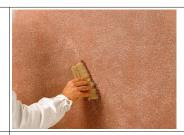
After a short flash off time the surface is spread/blended using a soft, dry wiper or brush to enhance the effect of bright particles.
