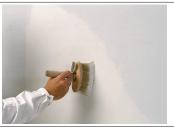
Brush applied priming coat (cross-coat) or intermediate coat if necessary.
